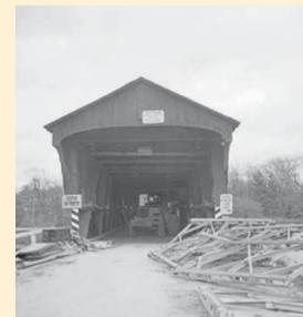
Bailey trusses, a type of portable prefabricated bridge, were added to the structure in 1959.
