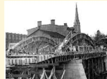
Construction underway on the 1931 concrete bowstring arch bridge.
