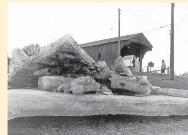
Ice jamming at the bridge during spring break up in 1981.
