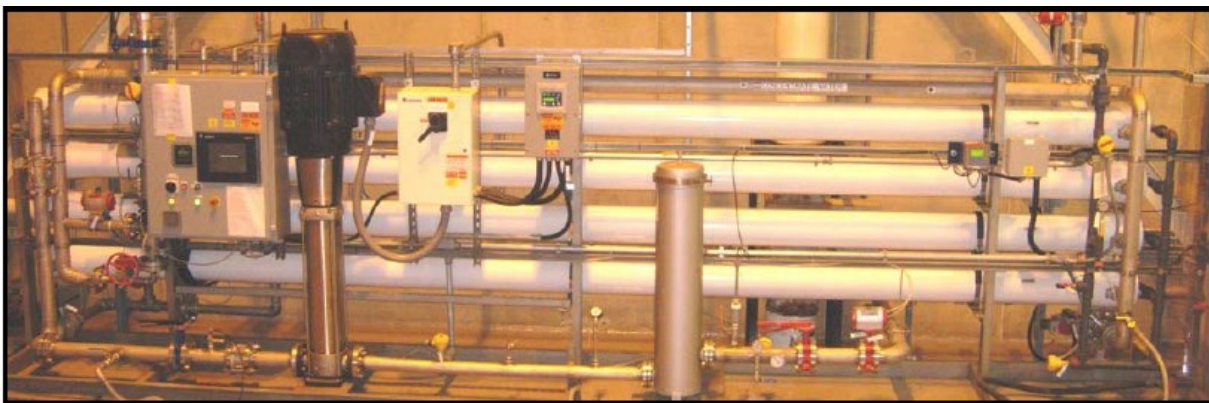
Figure 1 reverse osmosis concentrate recovery system
