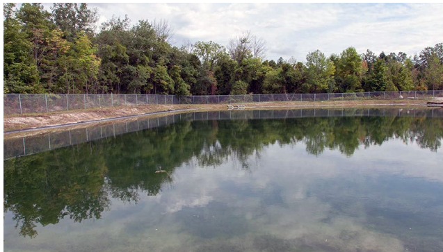
Figure 1 Chicopee Tube Park stormwater pond
