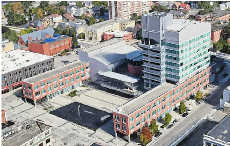
Figure 1 City of Kitchener City Hall
