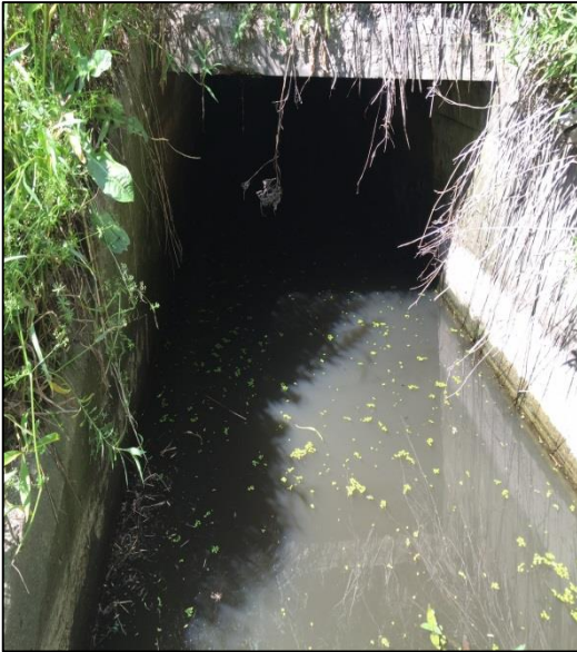
BD-ST3 Structure Inlet
