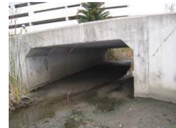
Forwell Creek flows beneath the railway north of Randall Dr.
