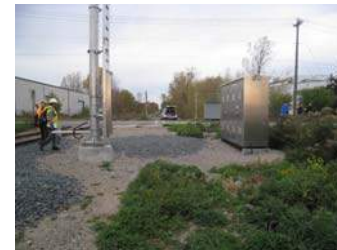
New railway infrastructure at Randall Dr.
