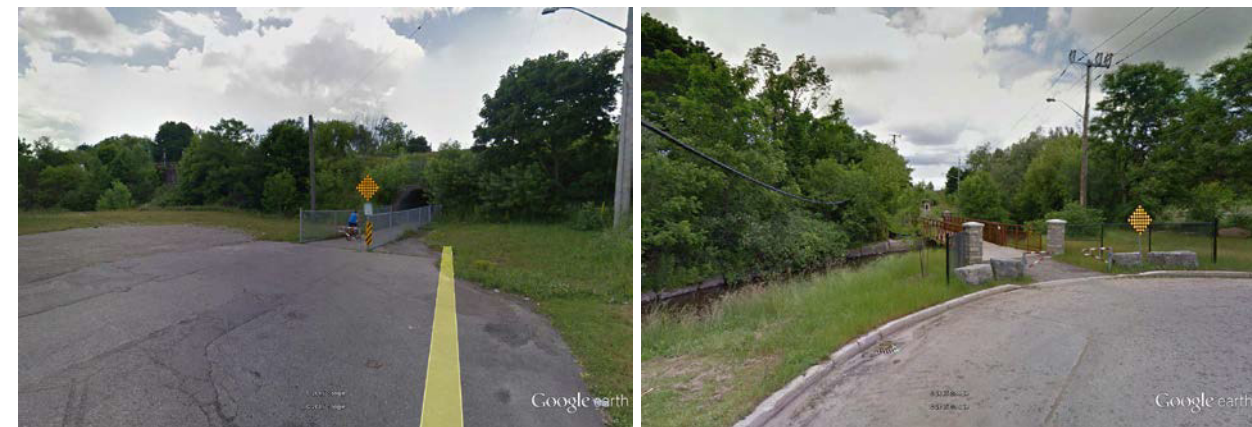
Figure 12: North/south sides of Elgin Street CP Rail grade separation
