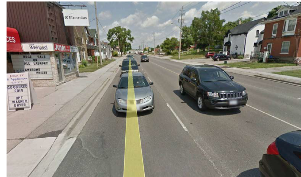
Figure 10: Water Street north of Dando Avenue (looking north)
