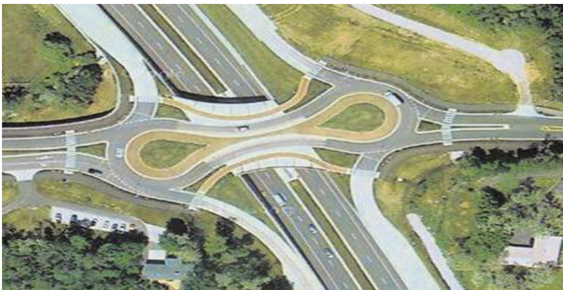
Figure 4A – Aerial Photograph of Bow-Tie Grade Separation Above 4-Lane Road
