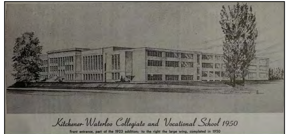
Front entrance, part of the 1923 addition; to the right the large wing, completed in 1950
