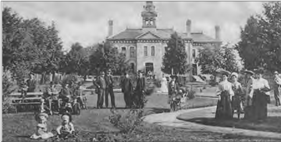
Preston Public School, 1905; Courtesy of the Toronto Public Library
