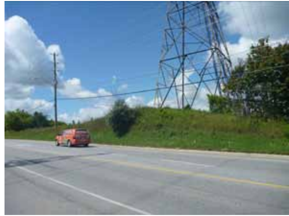
Plate 10: View northwest of study area. Erb Street ROW and Hydro Tower property are disturbed. No potential.
