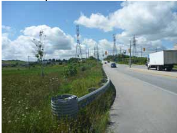
Plate 9: View southwest of Erb Street ROW. ROW is disturbed. Adjacent lands beyond ROW are low and wet. No potential.
