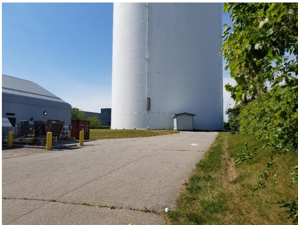
Image 3: View facing north at disturbances associated with the existing Pinebush Water Treatment Plant (PBTW1-10).
