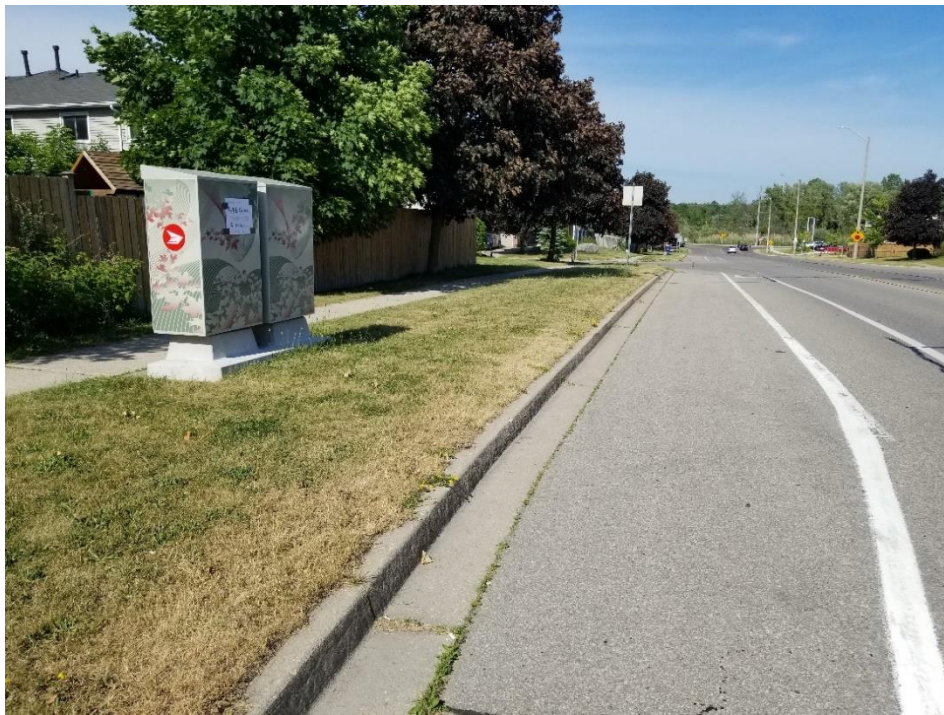
Image 14: View facing northeast at disturbances associated with the existing paved Saginaw Parkway and existing infrastructure (watermain construction along Saginaw Parkway).
