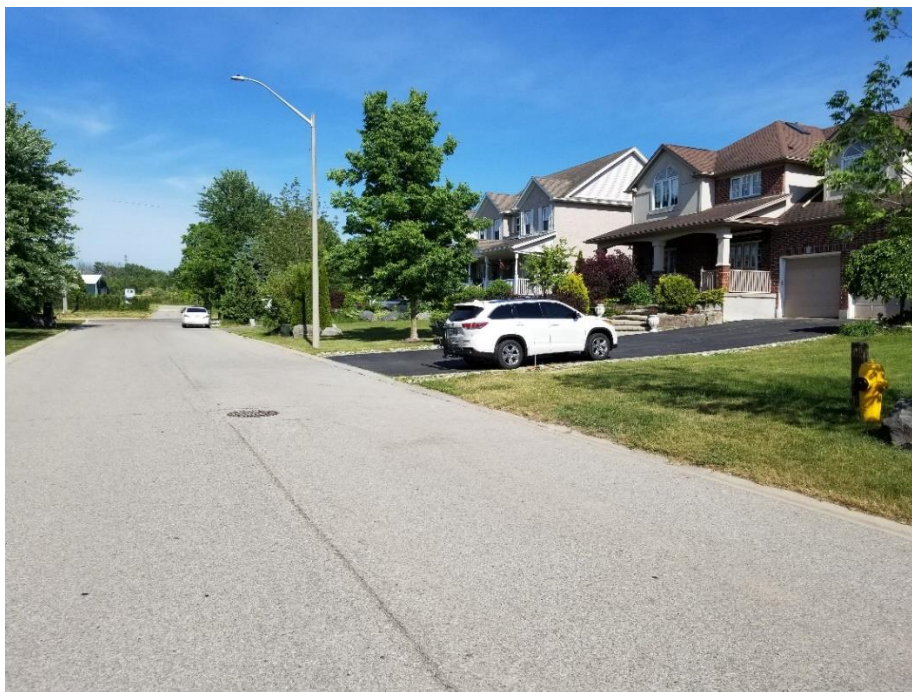
Image 10: View facing east at disturbances associated with the existing paved Cedarbrook Court and underground utilities (Cedarbrook well site and watermain construction).
