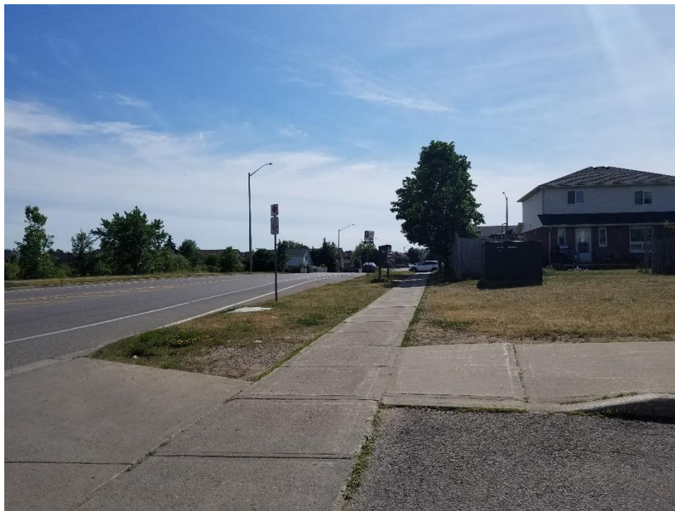
Image 16: View facing west at disturbances associated with the existing paved Saginaw Parkway and existing infrastructure (watermain construction along Saginaw Parkway).
