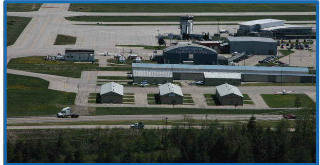
Image: Aerial View of Apron I
