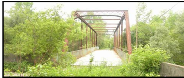
Nithvale Bridge, North Dumfries Township
