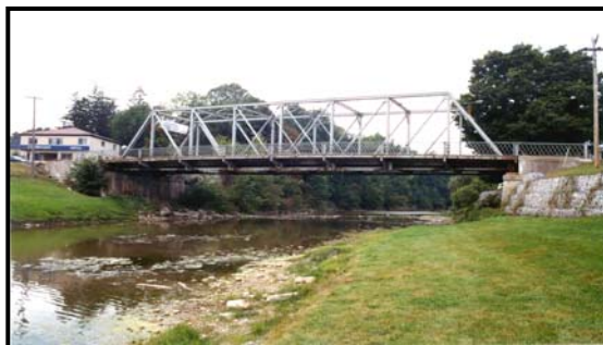
Hartman Bridge, Wilmot Township
