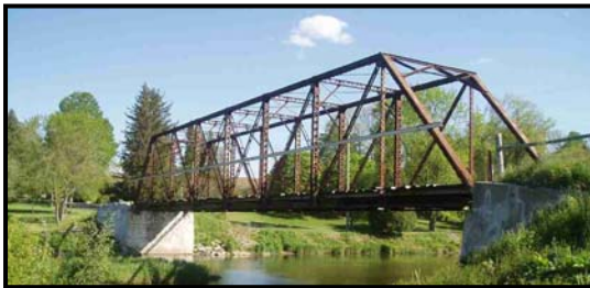
Piper Street Steel Truss Bridge, North Dumfries Township
