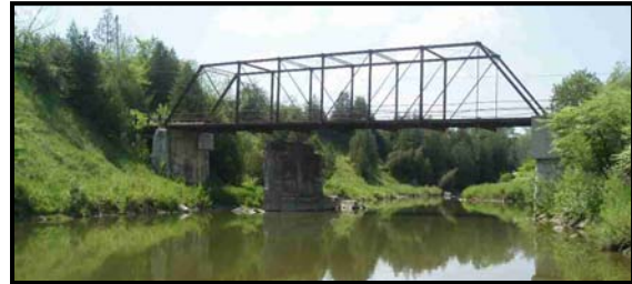
Wellesley Bridge #6, Wellesley Township
