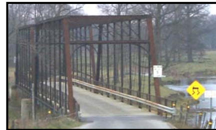
Conestogo Bridge, Woolwich Township
