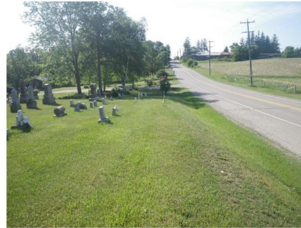
Image 6: View of the west side of the Old Portion of the cemetery adjacent to roadside ditching.
