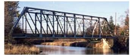
Haysville Bridge, Wilmot (Demolished)
