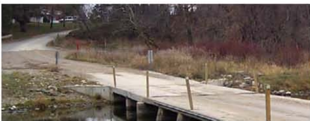
Mennonite Bridge, Woolwich
