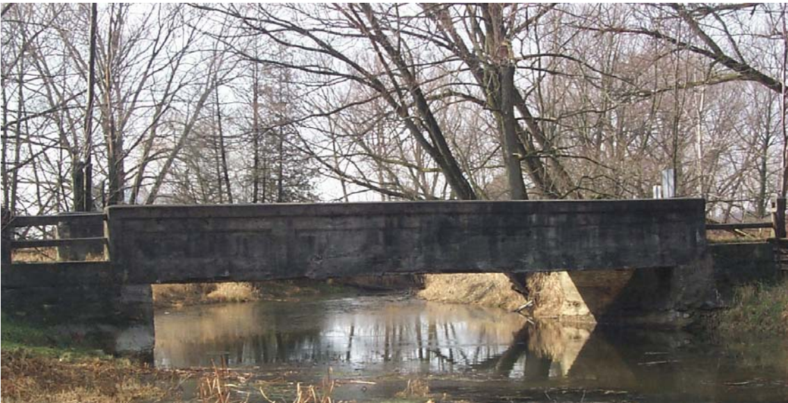
South West View
