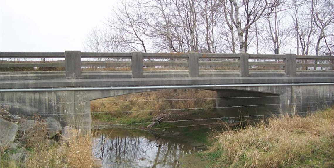
South West View
