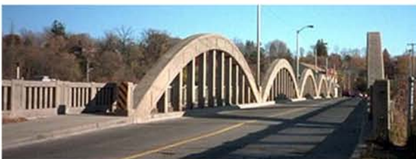
Bridgeport Bridge, Kitchener
