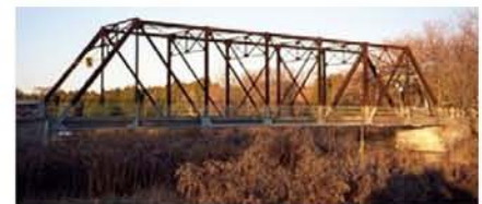
Blackbridge Road Bridge, Cambridge
