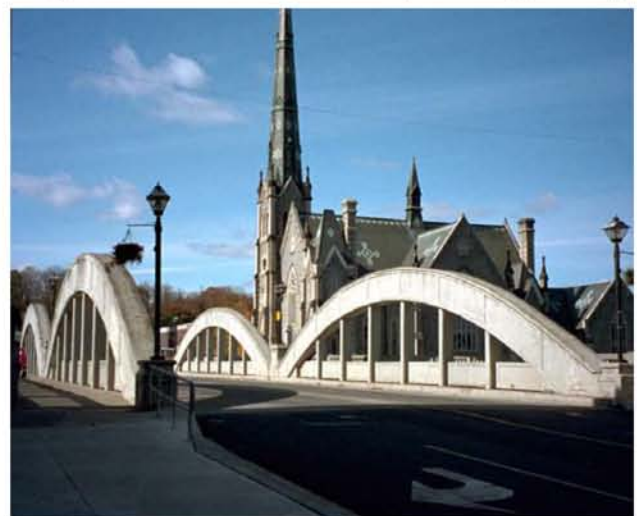
Main Street Bridge, Cambridge
