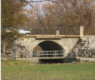
Mill Creek Bridge, Cambridge
