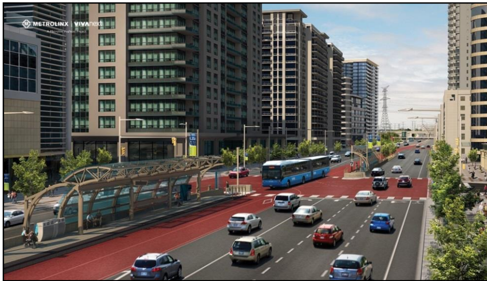
Figure 4-3: Staggered (Far Side) Side-Loading Platform Configuration (example from York Region vivaNext BRT)
